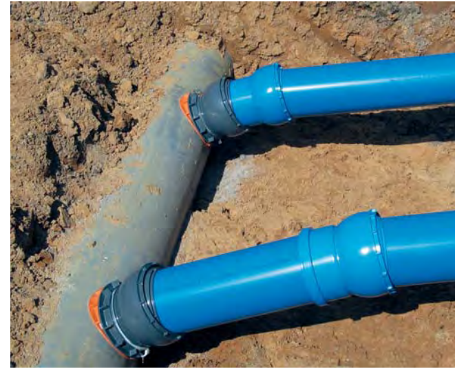
The perfect house connection: applying the HS-VARIO Coupler.
