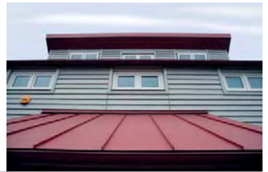
Partial view of the north façade with PVC window profiles.
