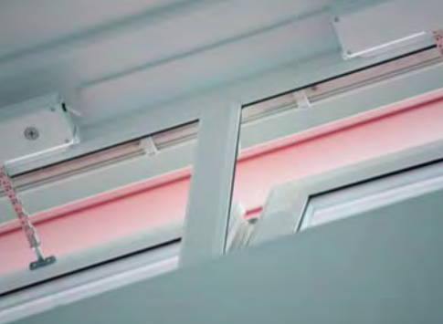
Automatic ventilation through the windows provides sufficient air circulation.
