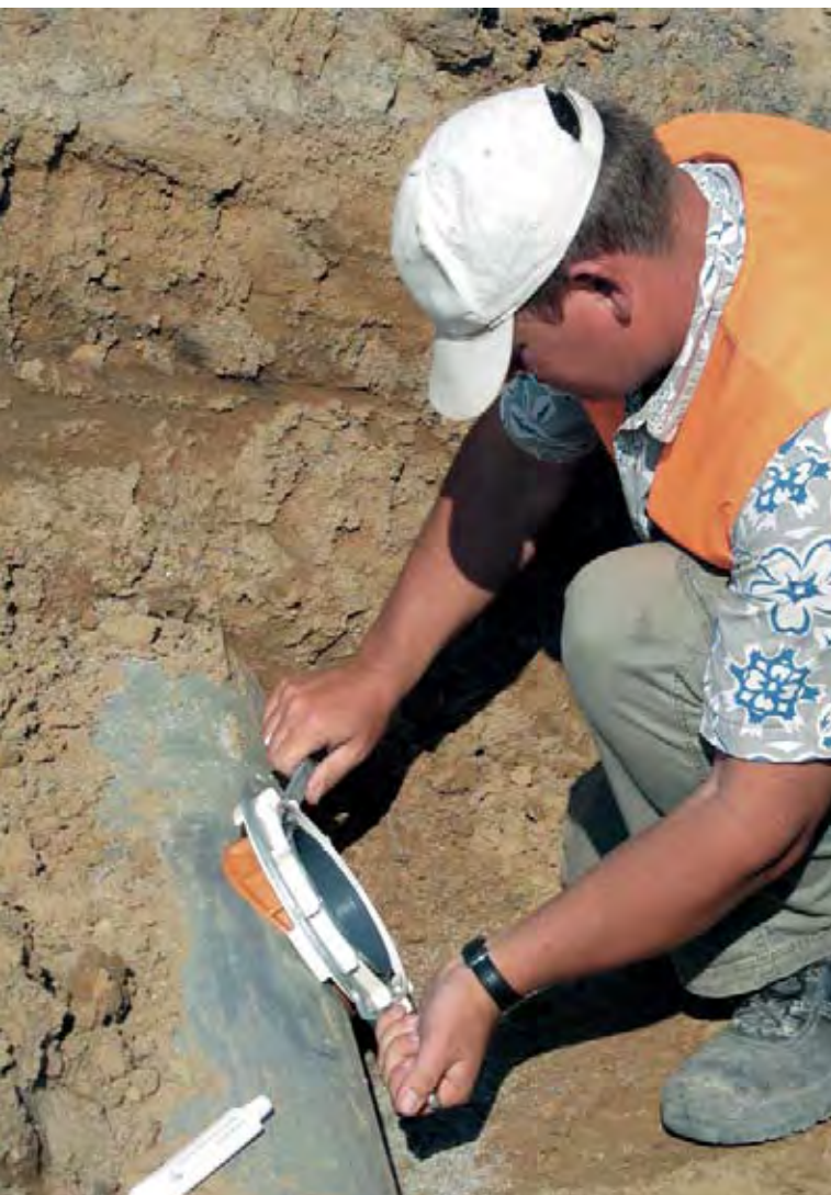
The house connections and lateral pipes can be joined quickly and easily to the main sewer through flexible fittings.
