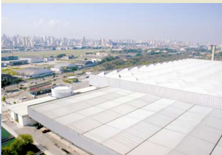
Pavilion at the Brazilian plastics fair "Brasilplast": The roof of the pavilion was completed with weather-resistant vinyl membranes joined with a layer of EPS.
