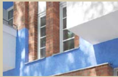
PVC window systems with the historically reconstructed sash-bars were used in the modernisation work in the 52 flats in Berlin-Neukölln in the style of the original façade.
