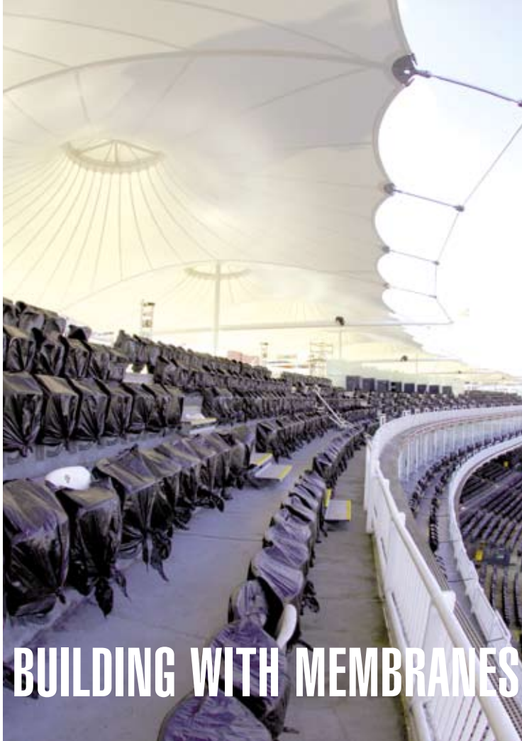
Left: View from below to the roof construction of the London cricket stadium with its impressive PVC membranes.
