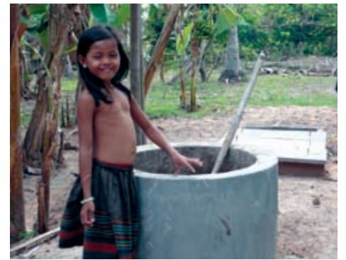
Future biogas user in front of a completed system.
