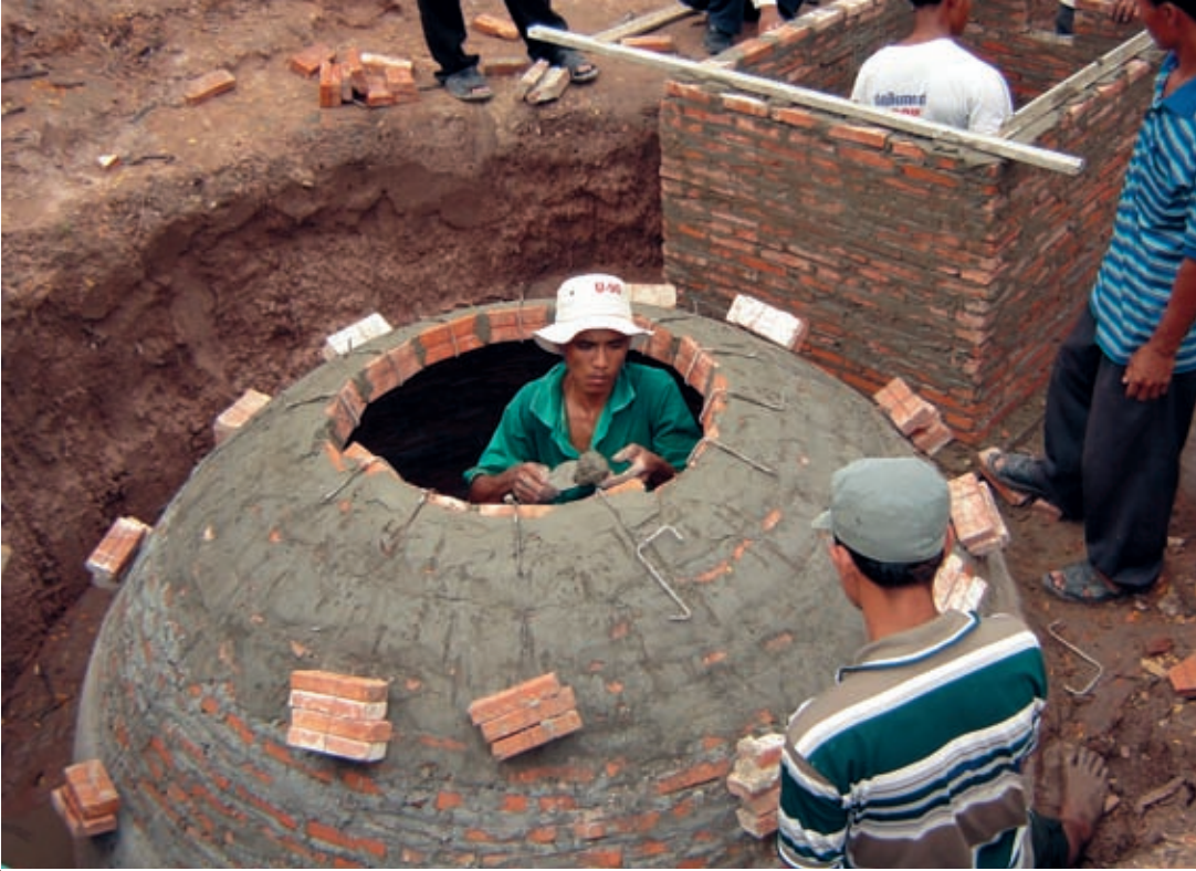
Bio-digester shortly before its completion.
