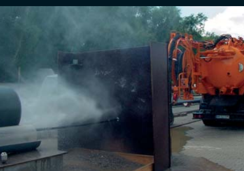
The water was forced through the pipes with up to 120 bar.
