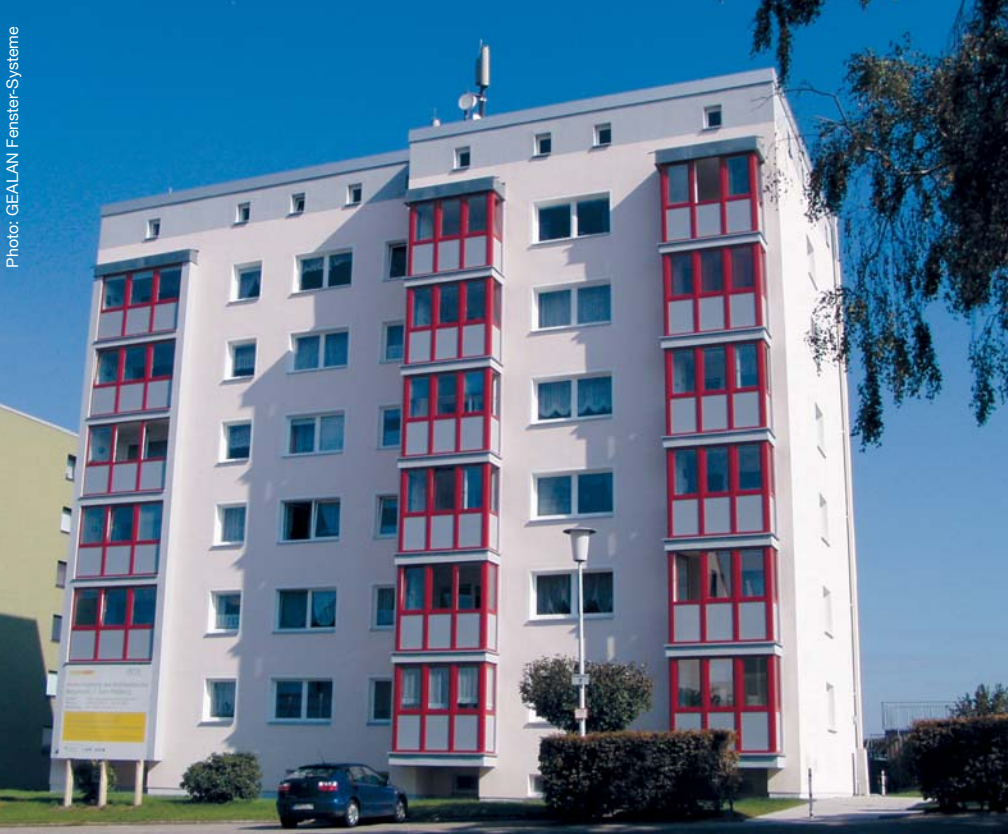
The energy-efficient improvements of this high-rise building in the German city of Selb-Plößberg reduced the annual primary energy needs of 401 kilowatt hours per square metre a year to 25 kilowatt hours.
