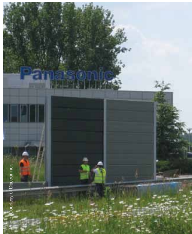
Sound barriers made of recycled PVC
